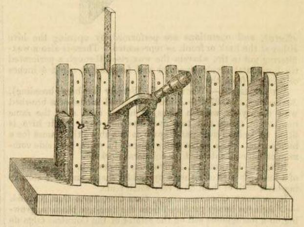
that the straw is subjected to pressure by means of a lever, and confined by means of iron pins passing though holes in the uprights. The binding or stitching is applied before these pins are removed, and the result is a straw fabric of great firmness and solidity. The extreme cold of German winters is provided against by these straw hives being 2 inches thick.
